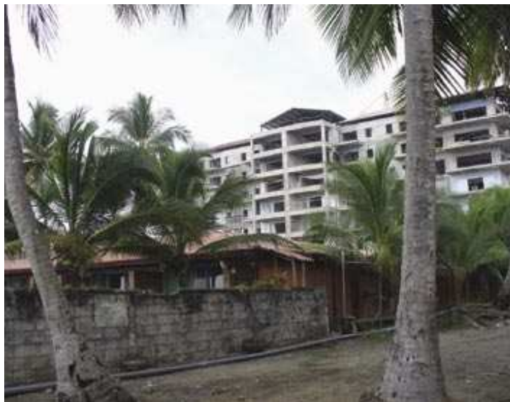
High-rise condominiums line much of the beachfront in Jaco. The population growth has fueled the construction of major commercial centers in the area; one just opened and two more are under construction.
